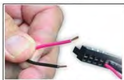
Strip each conductor 1/4"
