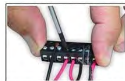
Place one wire at a time and tighten
